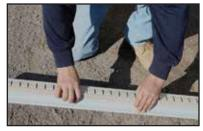
Make sure to join angles together with a coupler (6" piece of PVC).
